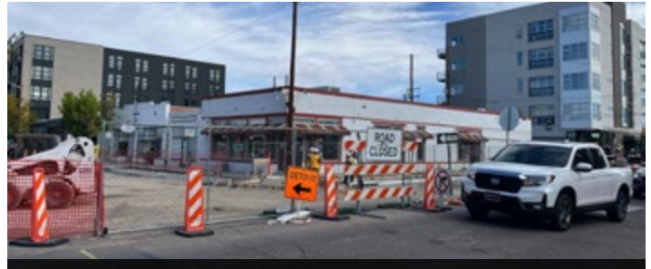
Construction impacting businesses on Louisiana and S. Pearl
